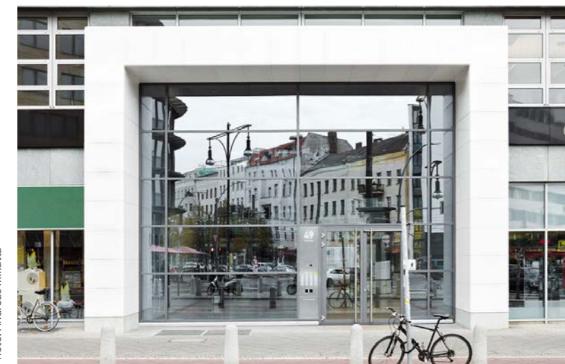
During the day, the lighting technology is invisibly hidden and protected by the robust HIMACS surface.
