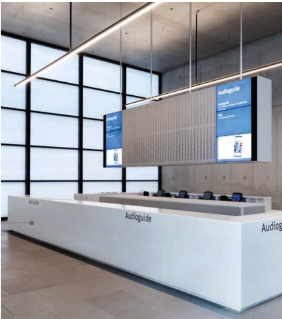
All of the counters in the new David Chipperfield building are constructed as solid, large-scale cubes. The design is made possible by the visually seamless craftsmanship of HIMACS.
